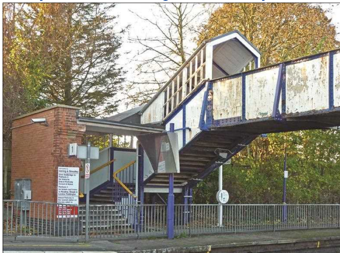
Old footbridge - platform 1 - 5 Nov. 2012
