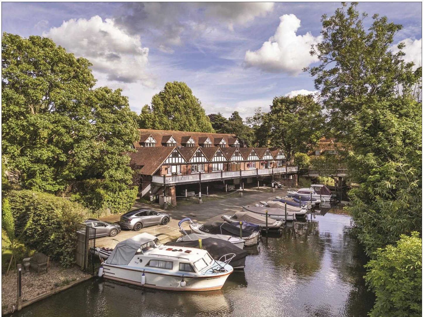
Saunders' Boathouse in May 2025 © Historic England Archive. See pages 5 and 43.
