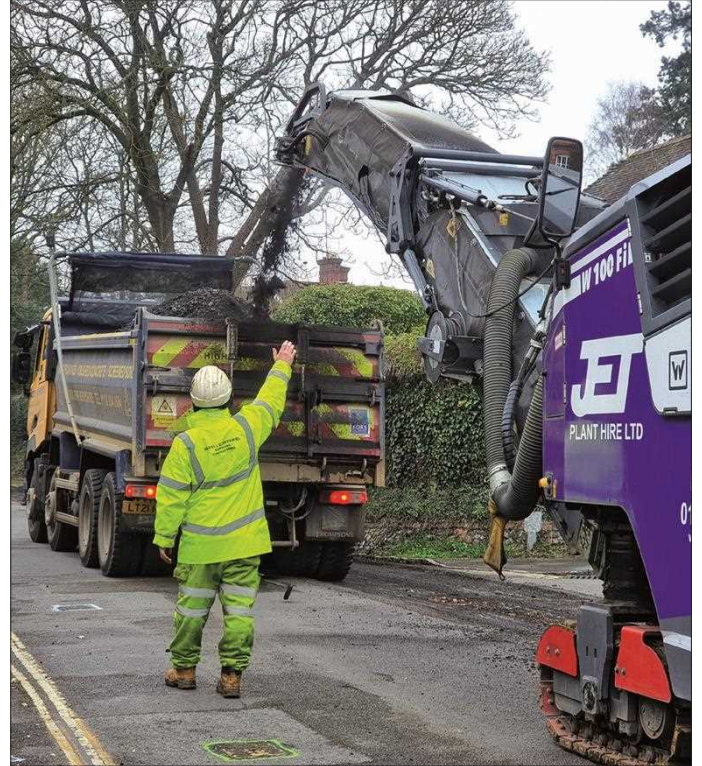
Pedestrian work on Station Road
