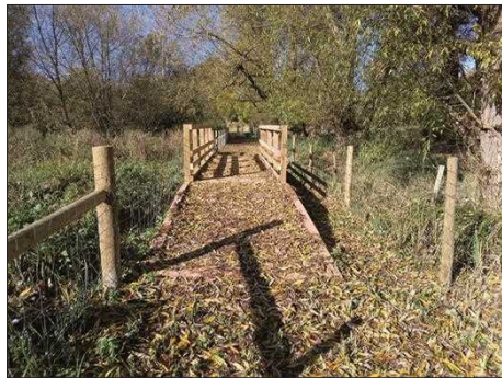
East meadow with new bridge - 5 October 2025
